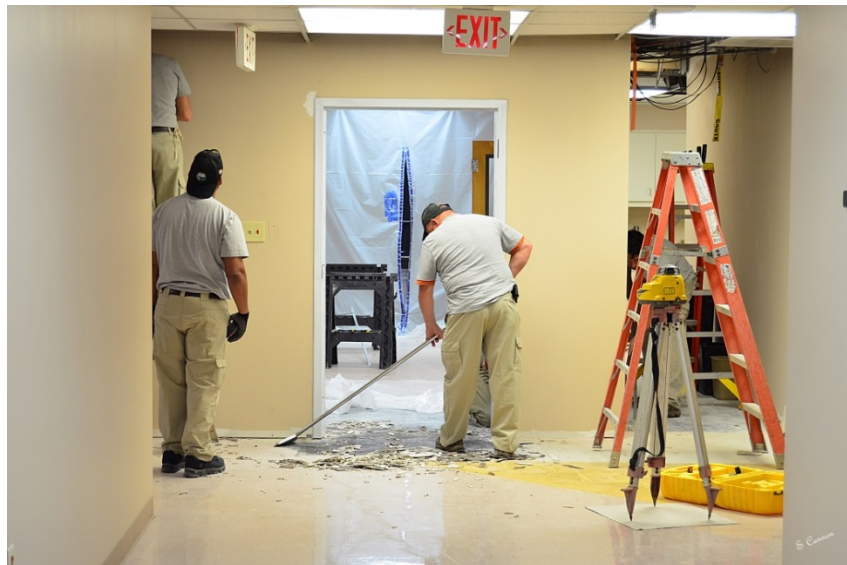
Facilities Maintenance personnel work on renovations to the McDaniel Building
