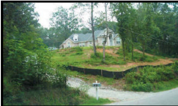
Perimeter silt fence with stabilization
