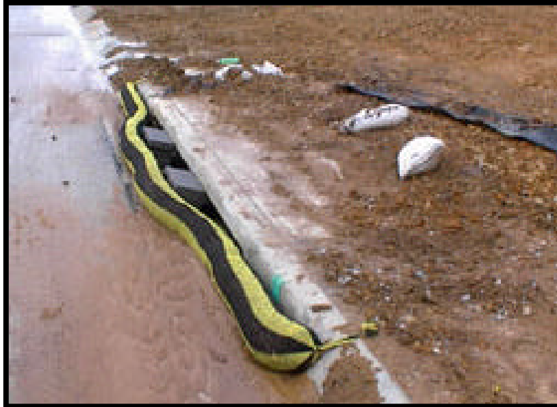
Photo 1 Compost Filter Sock Used for Inlet Protection
