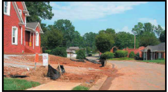
Poor construction entrance with 1/2" stone & tracking
