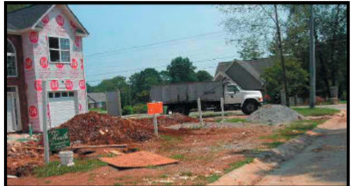
No silt fence causes tracking and erosion
