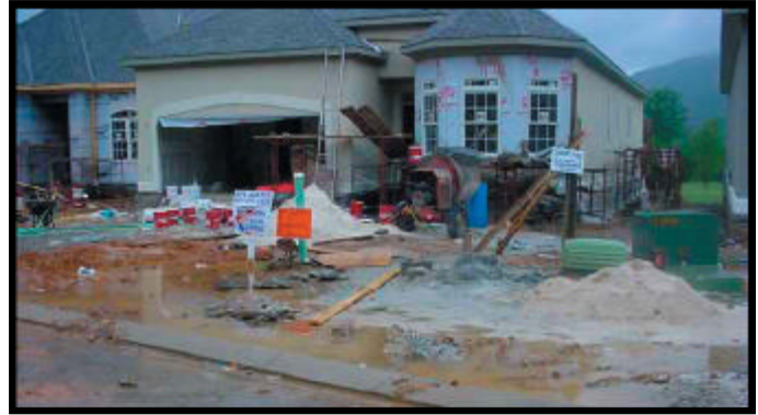
Parking on site damages property and tracks streets
