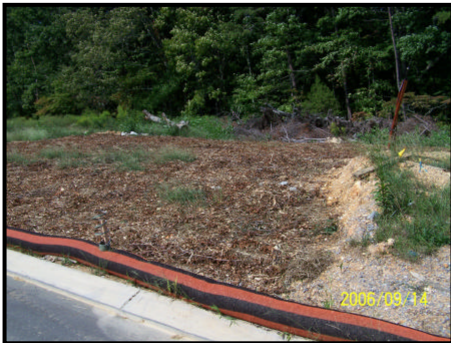
Photo 3-4 Compost Filter Socks- Installed
