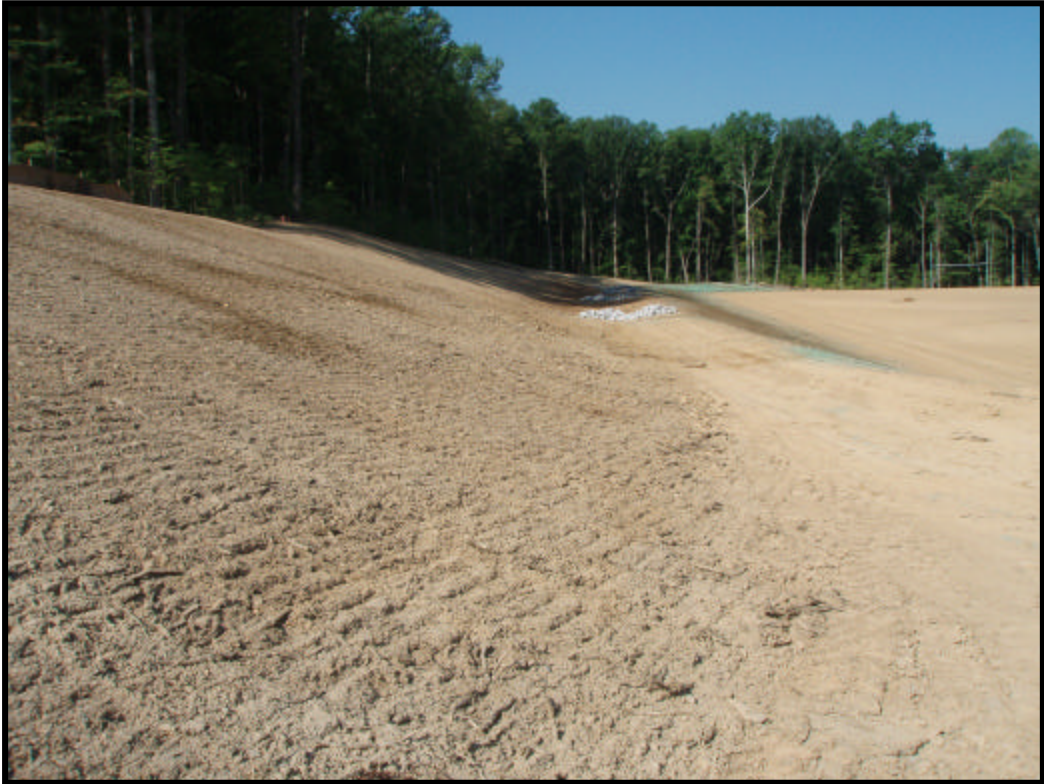
Photo Surfacing Roughening
