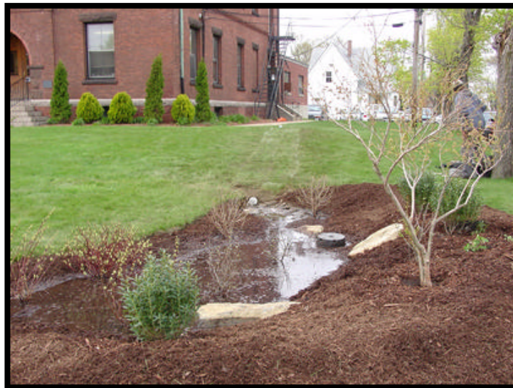
Rain Garden for Commercial Building & Parking Lot
