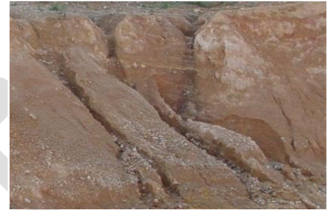
Severe Gully Erosion
