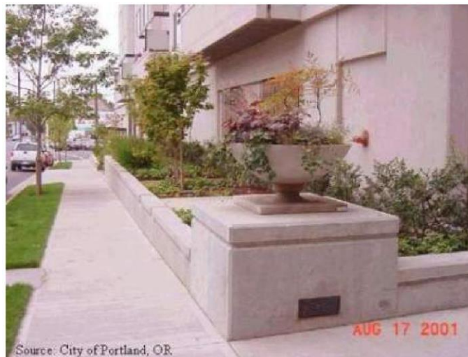
Figure GIP-02-01. Stormwater Planters (source: City of Portland, OR)
