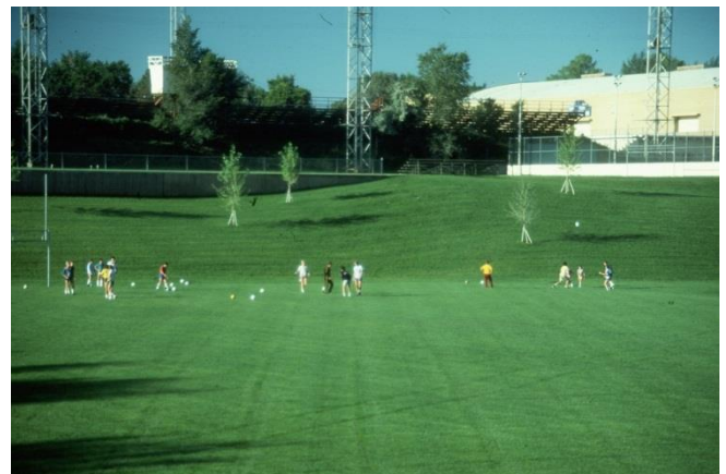
Figure GIP-06-02. Multi-Use Dry Detention Doubling as Sports Fields Englewood, CO
