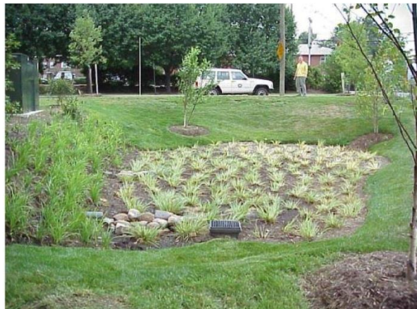
Figure GIP-01-01. A typical Bioretention Basin treating a commercial rooftop
