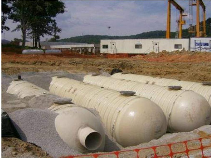
Figure GIP-11-12. Example of Multiple Fiberglass Cisterns in Series (Source: VADCR, 2011)
