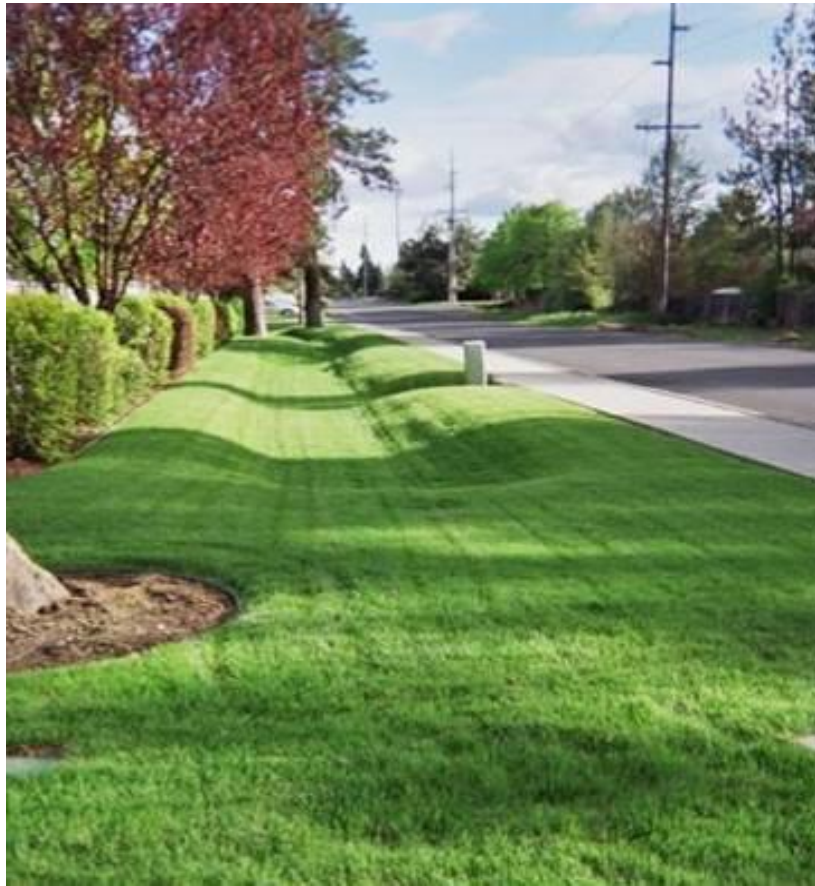
Figure GIP-08-06: Roadside Channel in Spokane, WA (VADCR, 2011)
