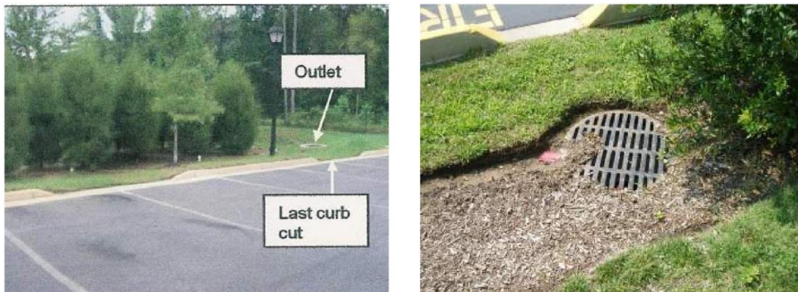
Figure GIP-01-08. Examples of Short-Circuiting at Bioretention Facilities (source: VADCR, 2010)
