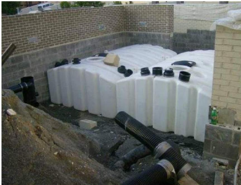
Figure GIP-11-13. Example of two Polyethylene Cisterns (Source: VADCR, 2011)
