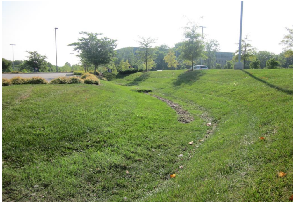
Figure GIP-08-05: Typical Grass Channel
