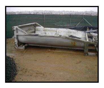
Photos 2 & 3 Self-Installed Washout Containers
