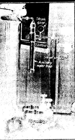
FIGURE 28—Steam-control assembly of air-space heating equipment.
